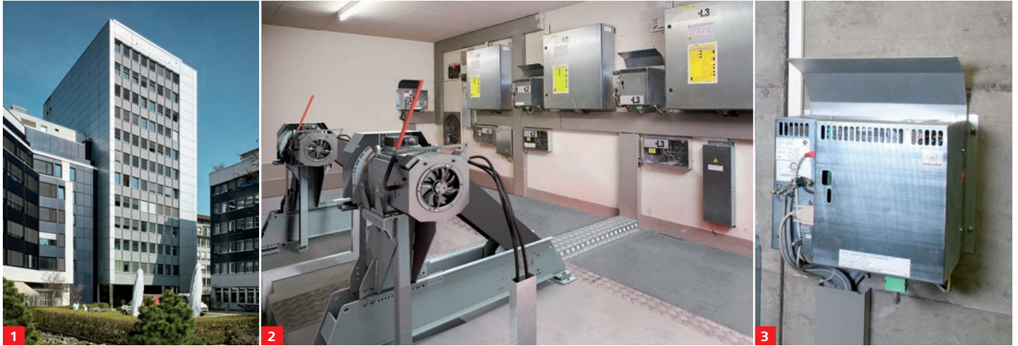
1: Typical building application | 2: Machine room | 3: Inverter with energy recuperation
